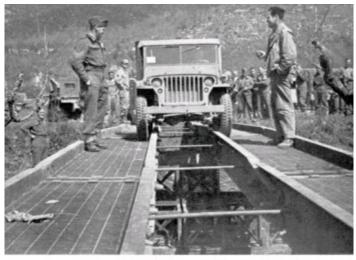
A jeep tests a Treadway bridge erected by New Zealand and American engineers in the Cassino area
